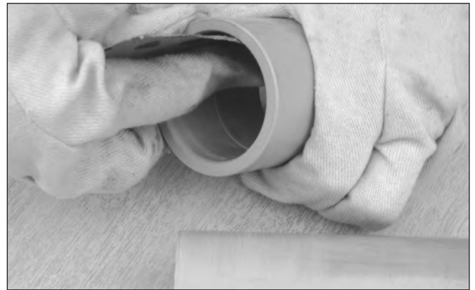
4. Abrade pipe and fitting.
