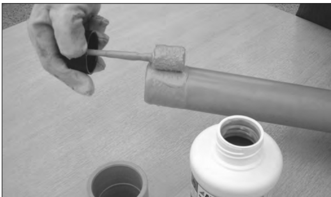
9. Apply cement to pipe and fitting.
