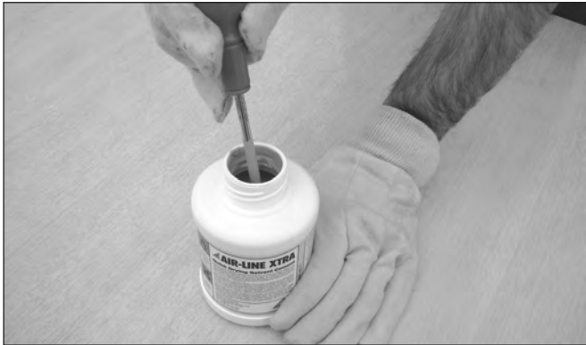
8. Stir solvent cement.
