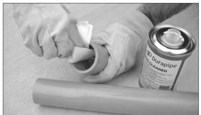
7. Clean pipe and fitting with eco cleaner.
